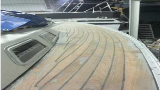
Fig. 19 Ready for mounting the fitting
